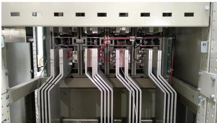
RTD connection in Busbar
