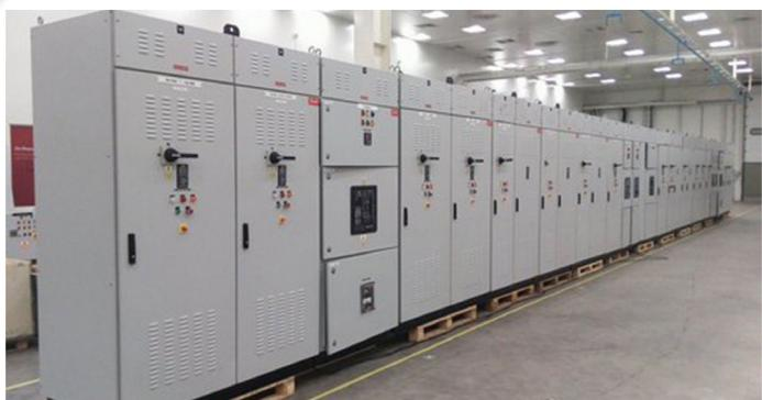
PCC PANEL / SWITCHGEAR PANEL
